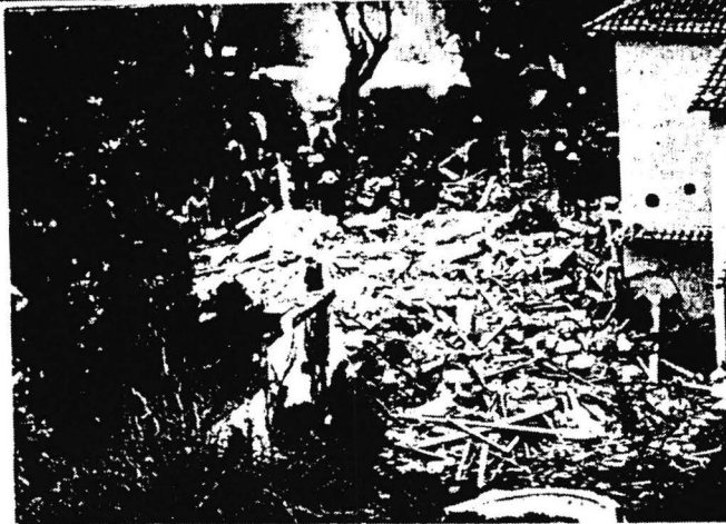
• An aerial view of the remains of Klein's house after the bombing early yesterday morning. (NA photo)
